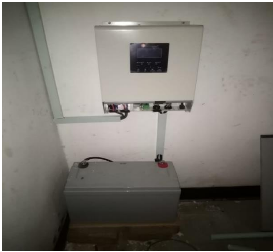
Fig. 3. 1kVA Inverter-battery backup system during installation inside Bank of Khartoum ATM service room
